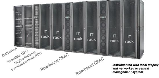
The data center system of **Figure 3** exhibits a 40% decrease in electrical consumption when compared with a traditional design, with the reductions in losses further classified as shown in **Figure 4**.
