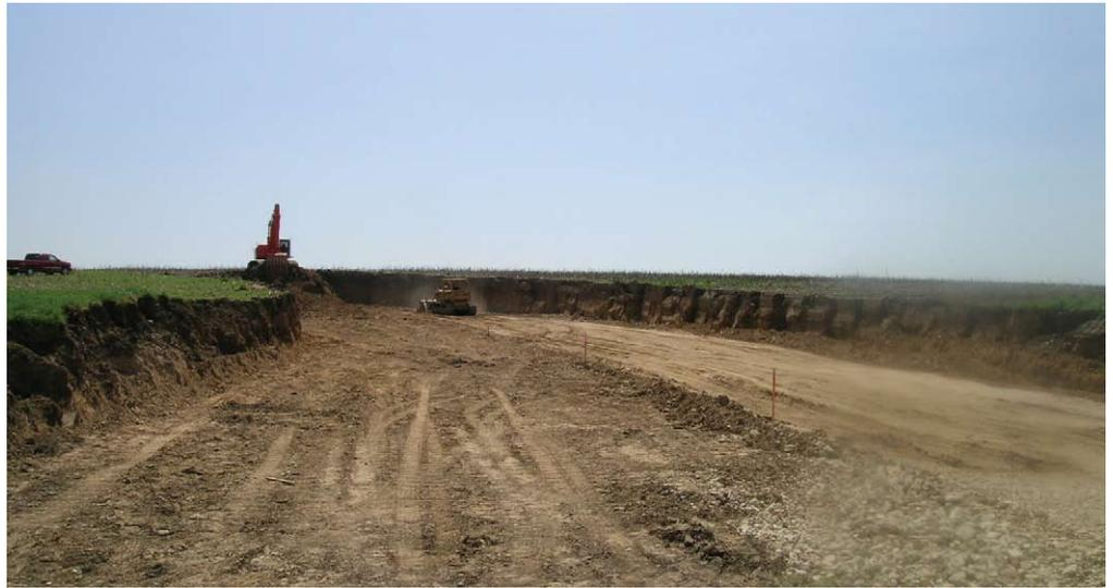
reconstruction of a 900-foot portion of an existing rural street to a 43-foot-wide urban section. The project also included design and construction of water mains and services, sanitary sewers, storm sewers, and sidewalk on one side. “The earthwork entailed some fairly significant cuts, and we had a really short time frame to get the design work done. In fact the whole project—from concept to bid—was only six weeks,” says Flesch.
